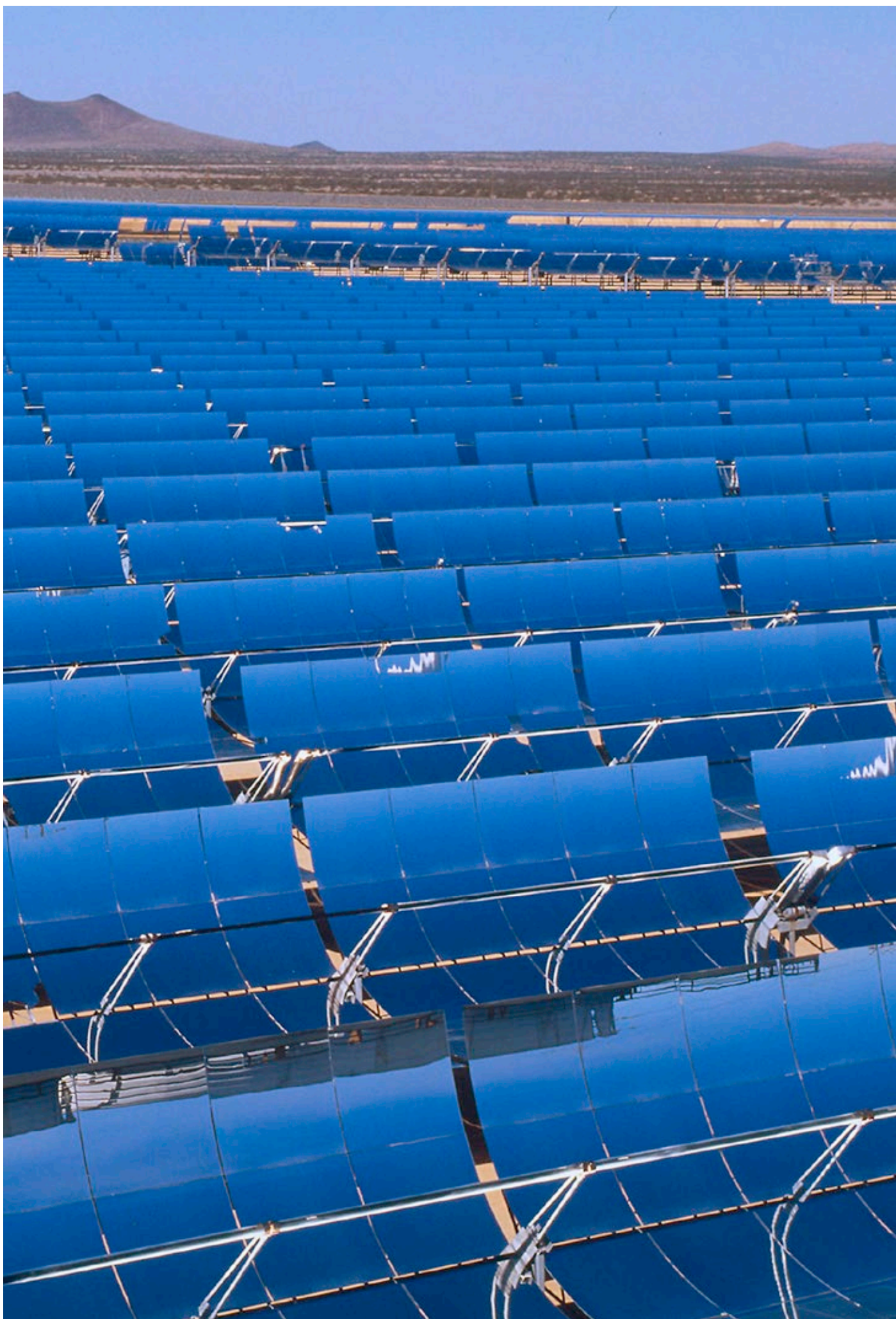
The world's largest solar power facility, named Solar 2, which produces 10 megawatts of electricity. The 1'926 heliostats provide 81'400 square meters of sun-capturing surface area. Daggett, near Barstow, California, Mojave Desert, United States of America
